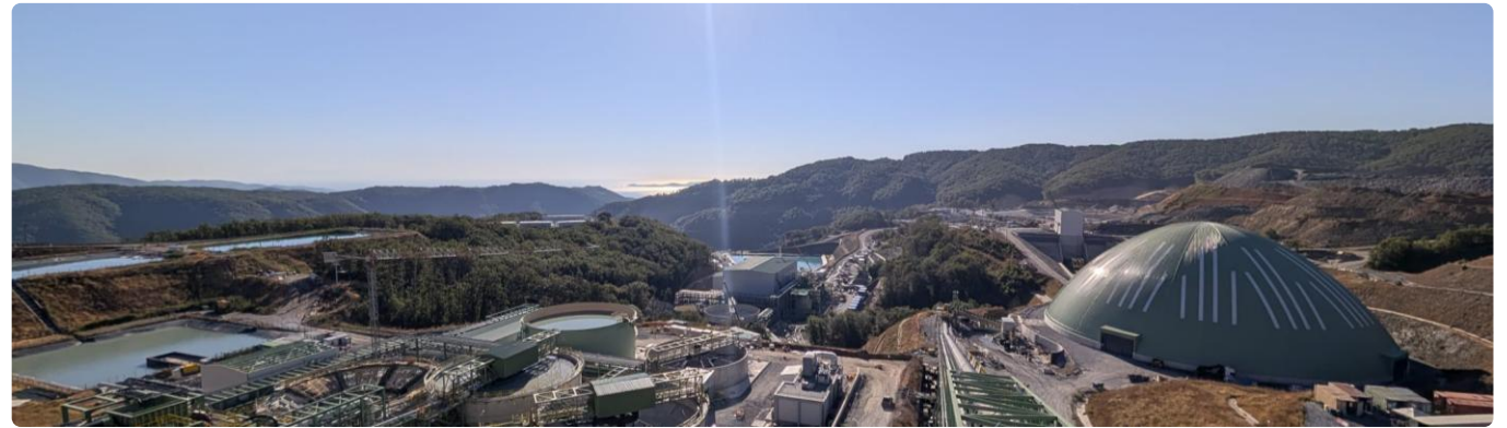
View from transfer tower
