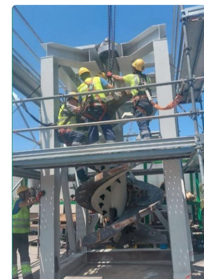
Verti-mill installation works
