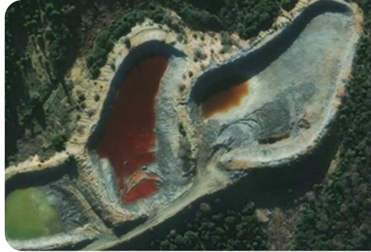
Before restoration work (2012)
