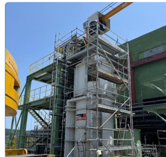
Verti-mill installation works
