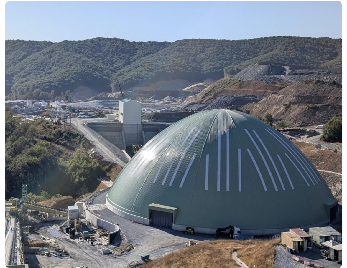
Dome and reclaim feeder, and SAG feed conveyor
