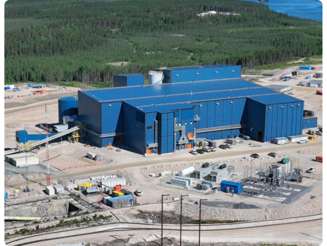
McIlvenna Bay - Aerial
