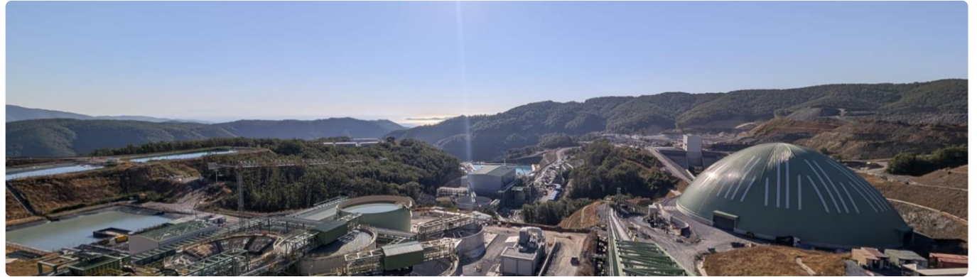
View from transfer tower
