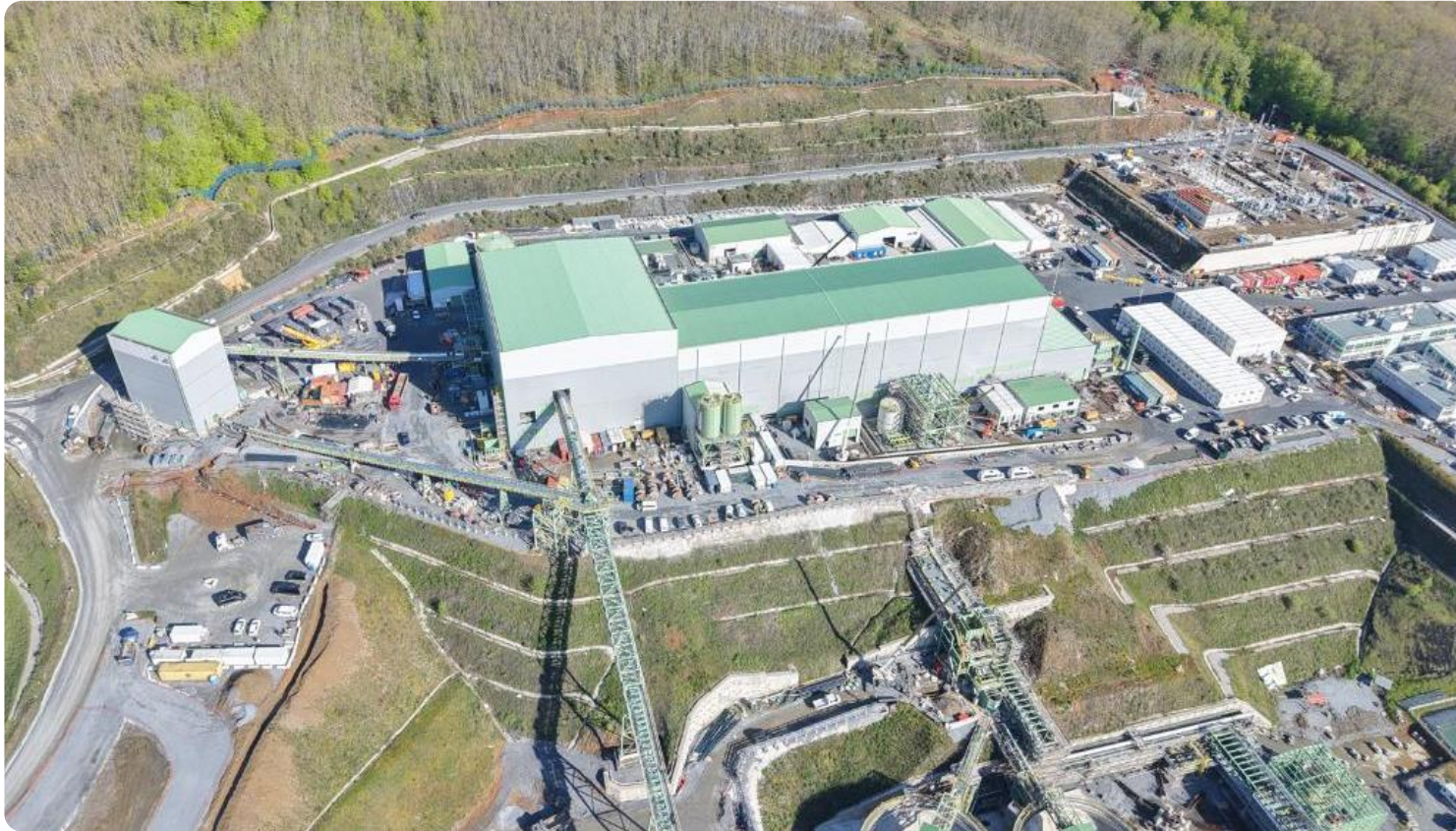
Aerial – process plant
