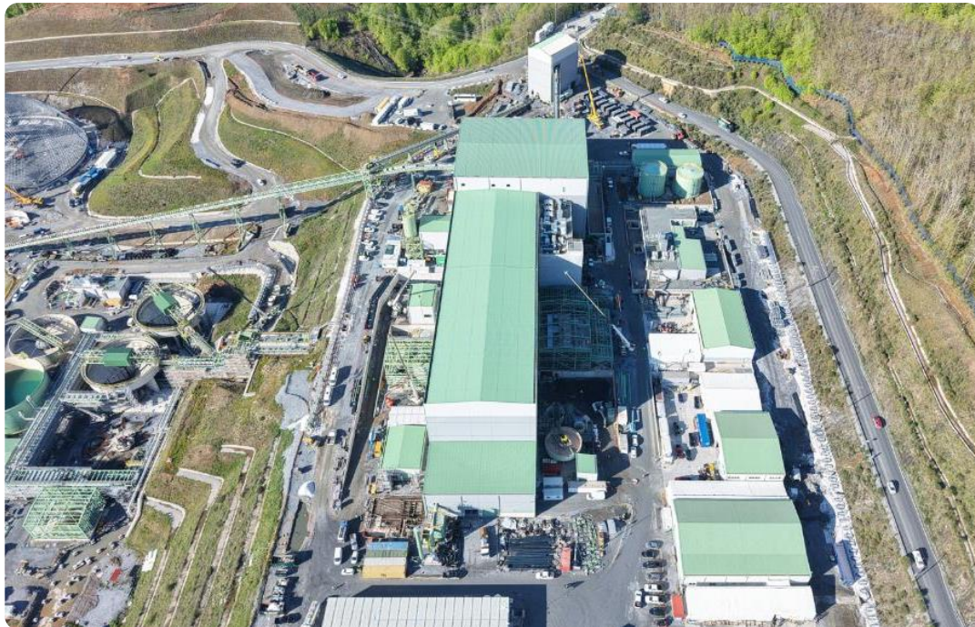
Process plant overview
