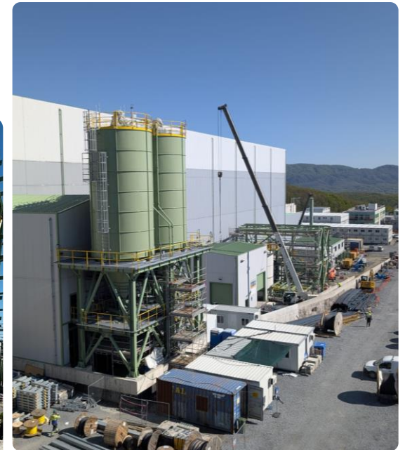
Lime, blower, guar and compressor buildings
