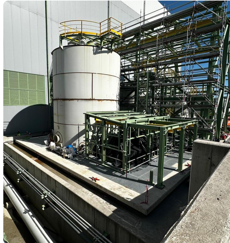
Guar building and tailings pipe rack
