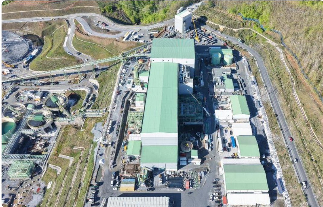
Process plant overview
