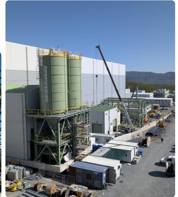
Lime, blower, guar and compressor buildings
