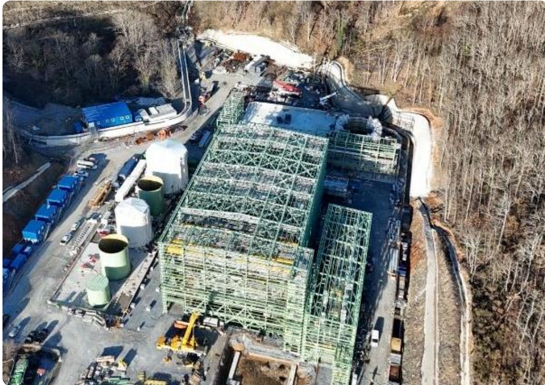
Filtered tailings plant overview, with tank farm progressing on the left and the compressor building on the right
