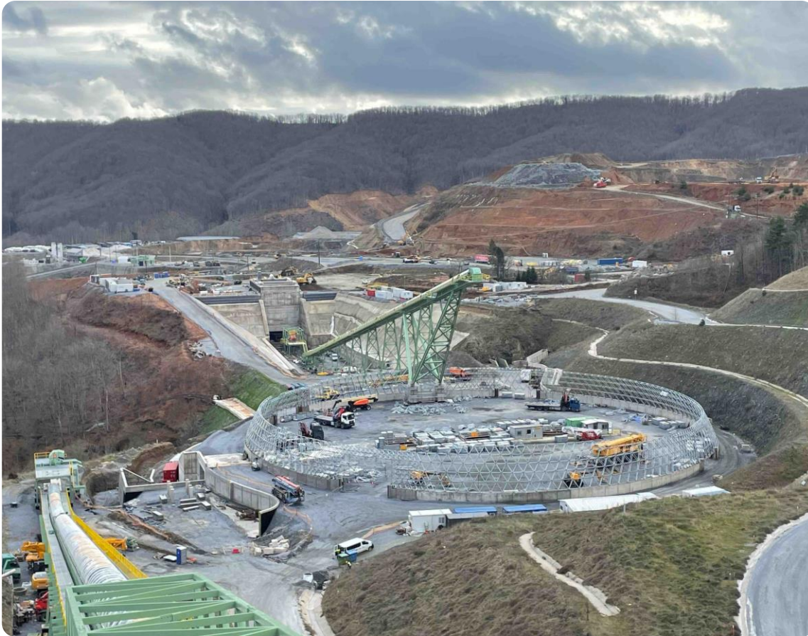
SAG feed conveyor and coarse ore stockpile dome
