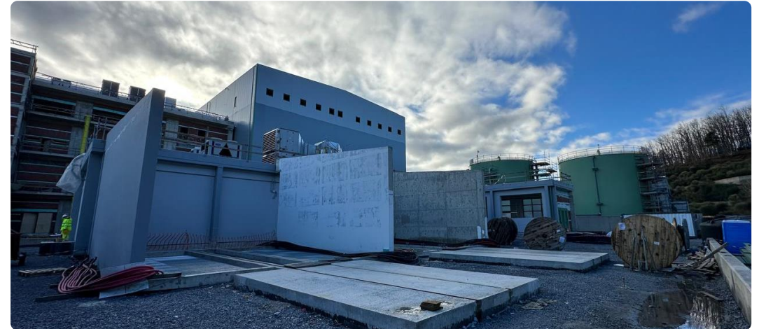
Substation transformer bays
