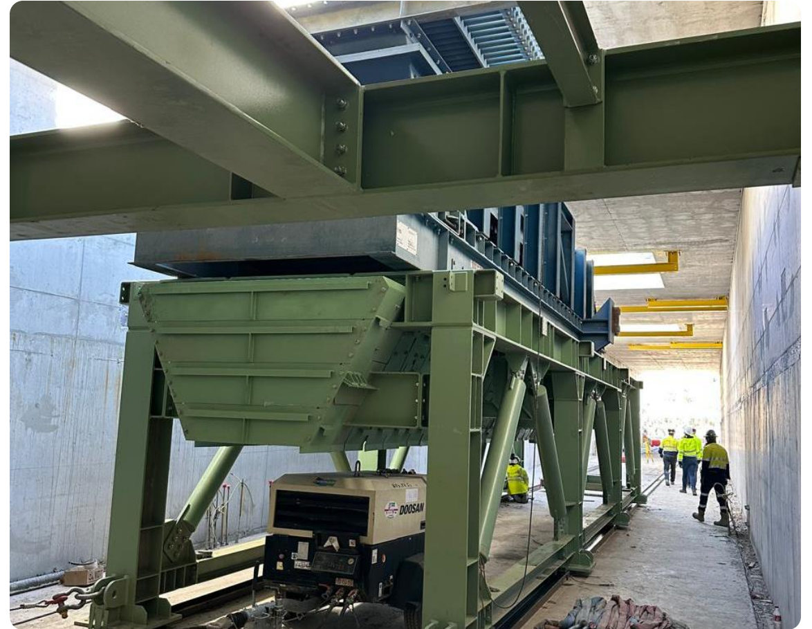
Reclaim feeder and discharge chute
