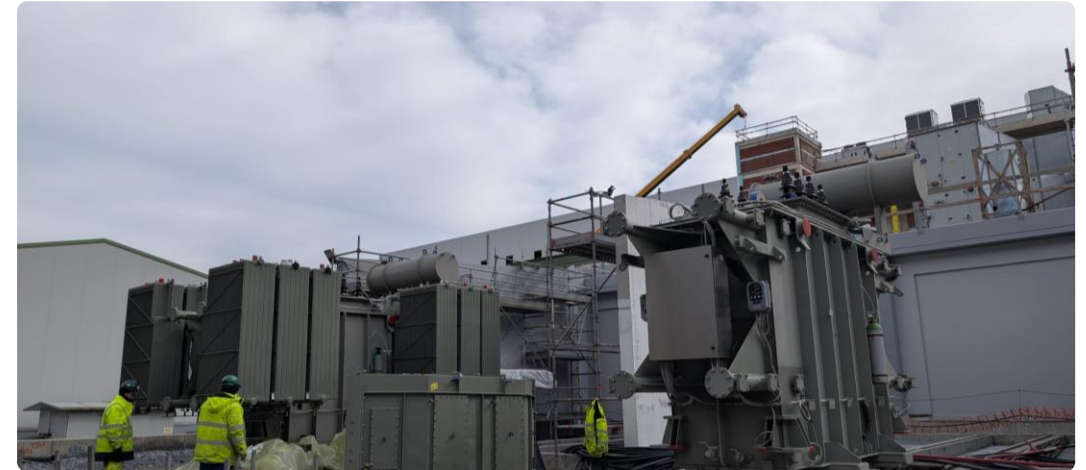
Substation transformer assembly
