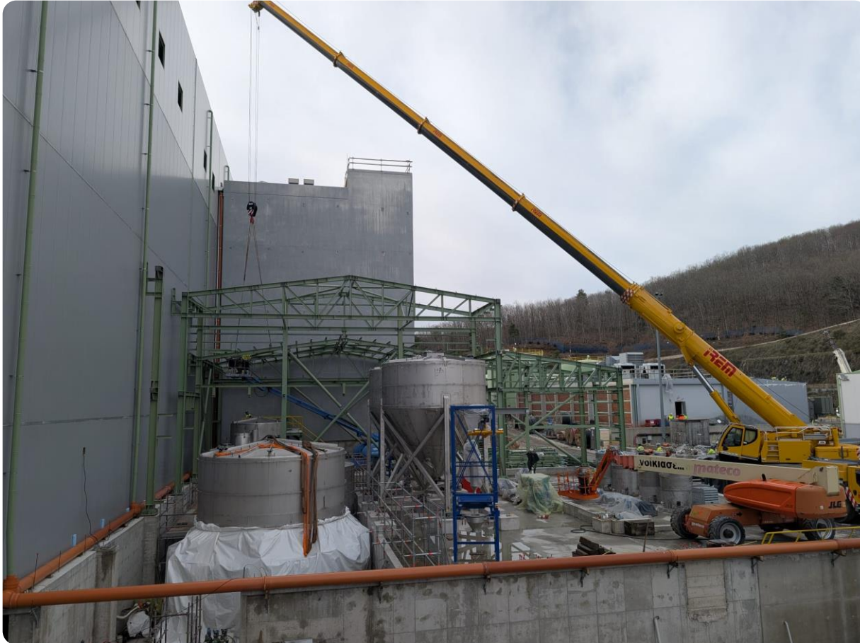
Sulphidizer building stand up and tank rough set
