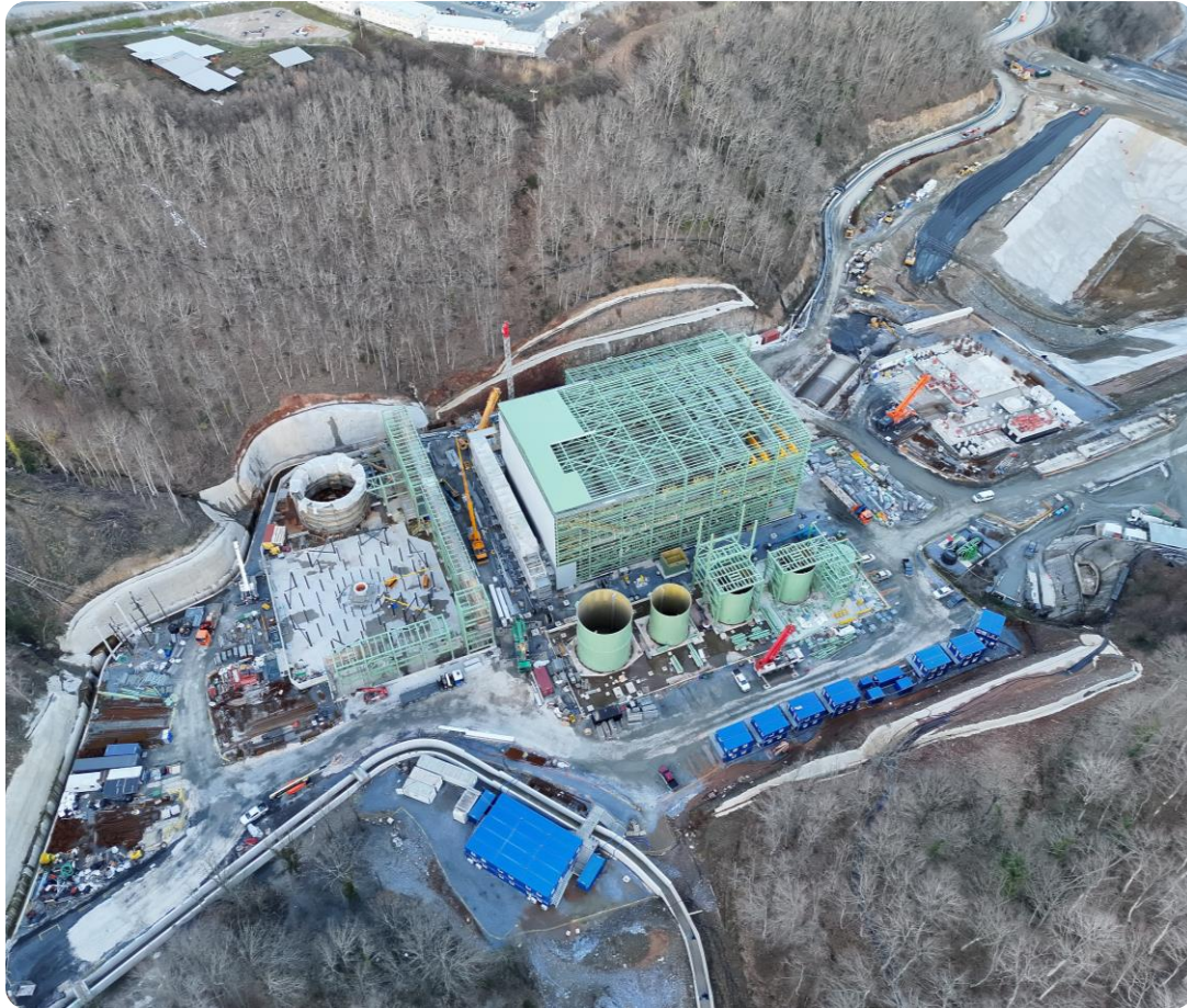
Filtered tailings plant overview, with tank farm progressing shown in front and the foundation of the compressor building on the left
