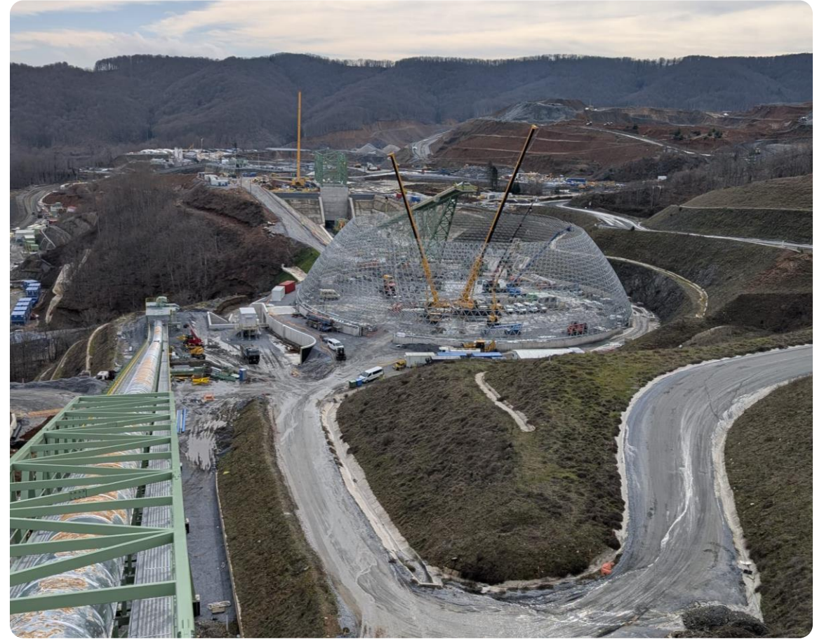
Dome and reclaim feeder
