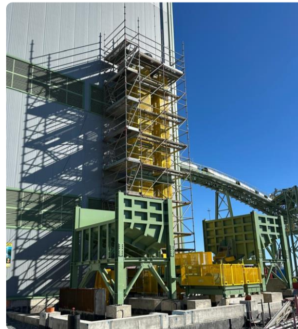
Mill media addition system
