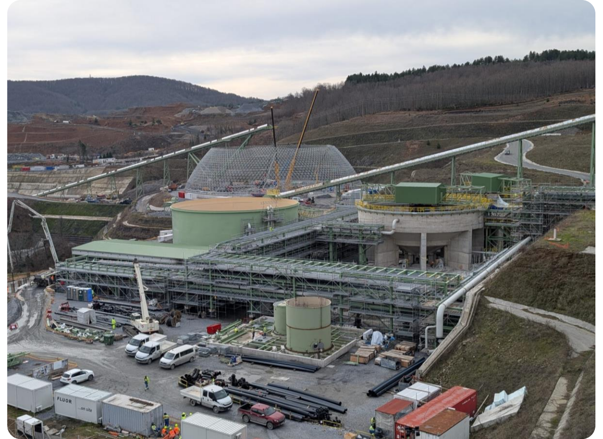
Tailing thickener pipe rack and distribution box
