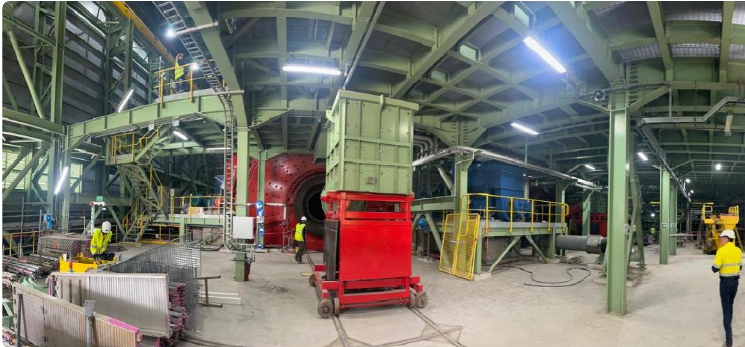
SAG & Ball Mill pre-commissioning activities
