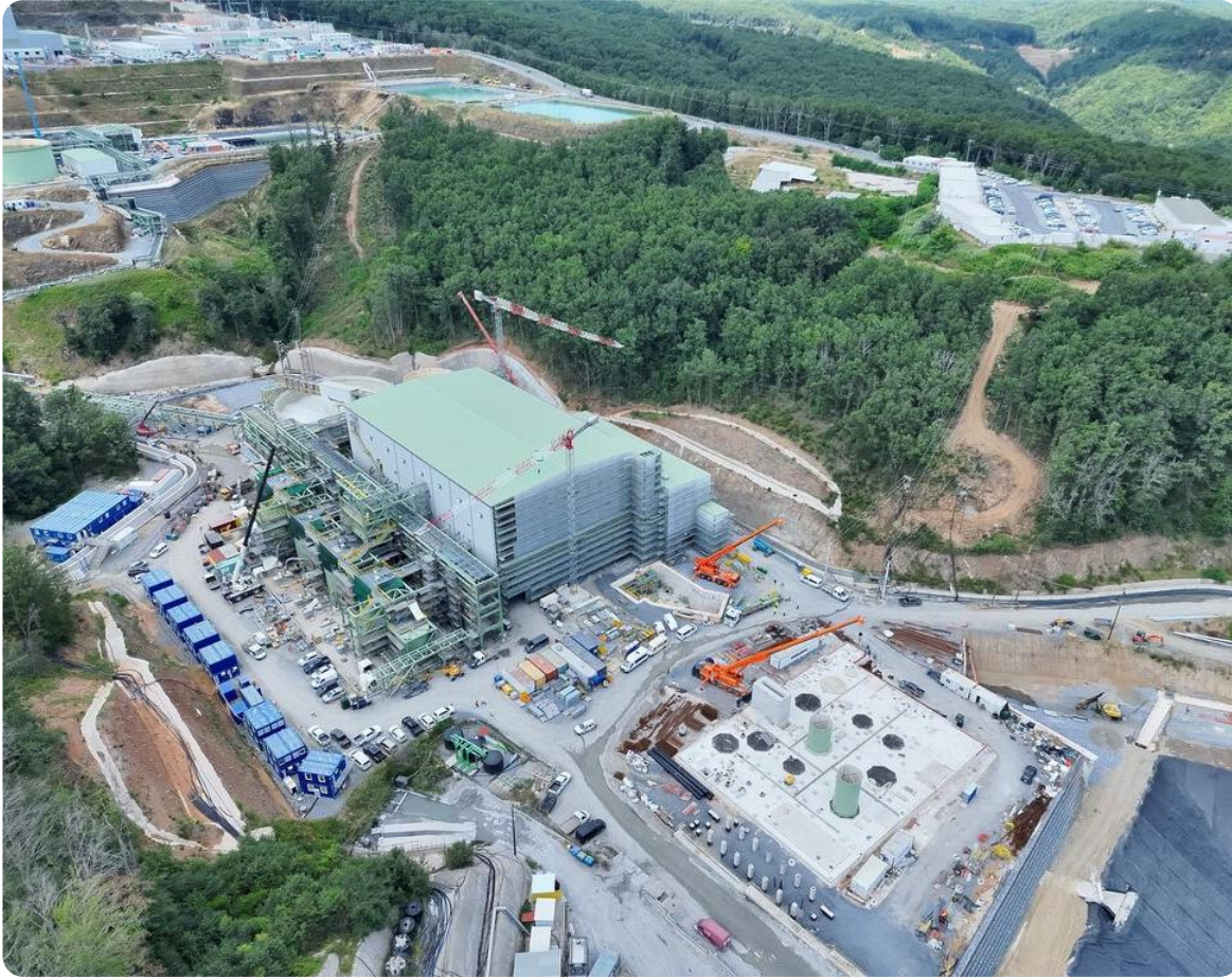
Filtered tailings plant overview
