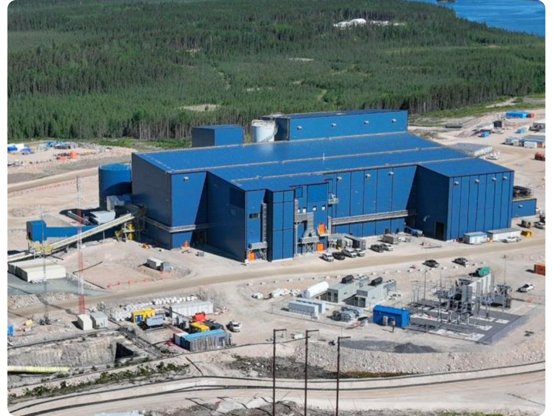
McIlvenna Bay - Aerial
