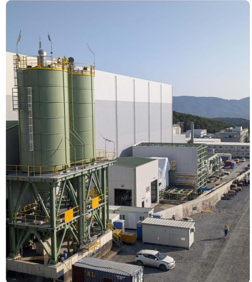
Lime, blower, guar and compressor buildings
