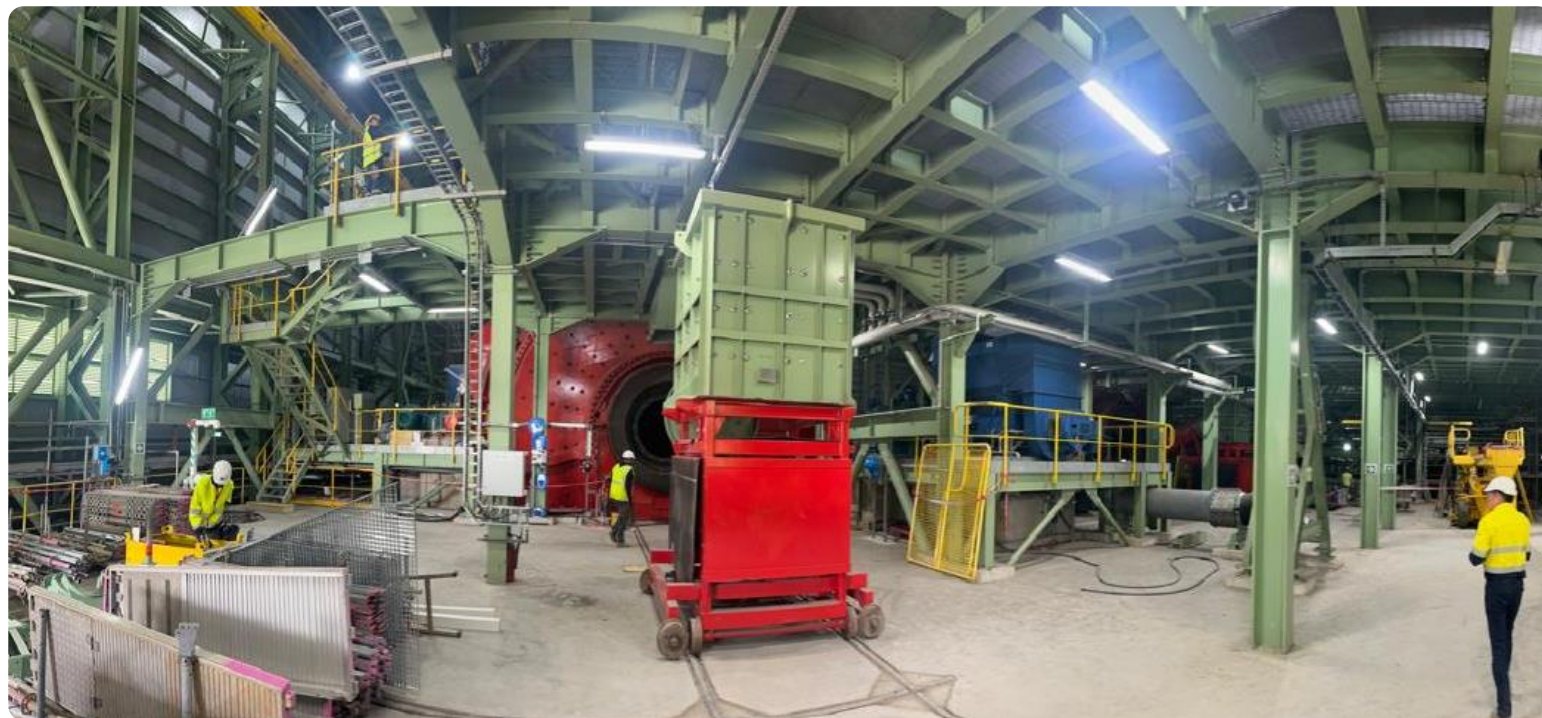
SAG & Ball Mill pre-commissioning activities
