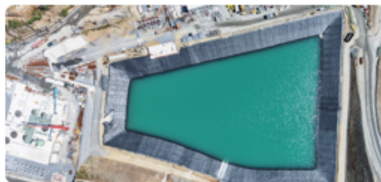
Water Management Pond #2 (Right) and Water Treatment Plant (Left)
