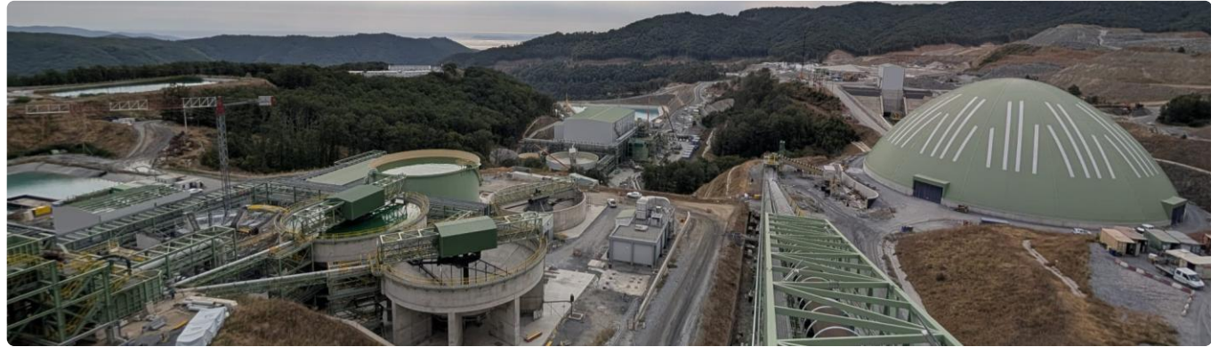
View from transfer tower
