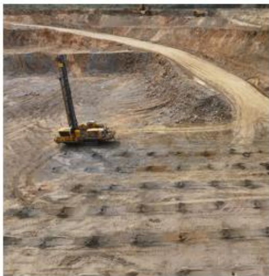
An autonomous drill advances across a bench at Skouries, creating evenly spaced blastholes to support consistent, high-precision blasting performance
