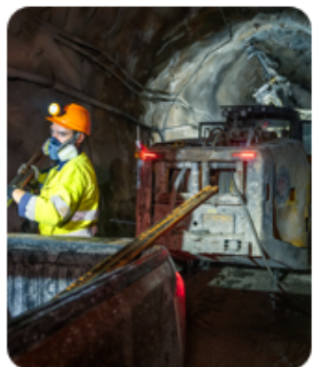
Drilling commenced with Trade Union Support
