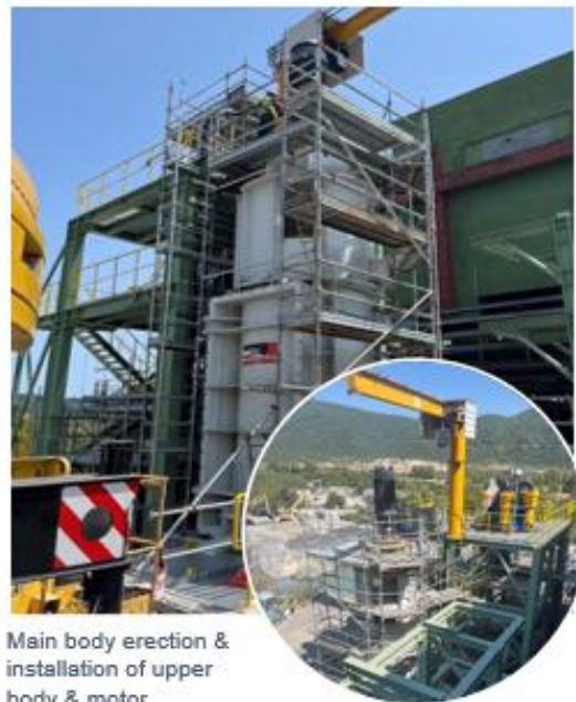
Mechanical works for Pb flotations cells 54 & 55 and Zn flotations cells 56 & 57
