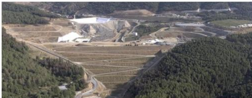
Kokkinolakkas Filtered Tailings Facility
