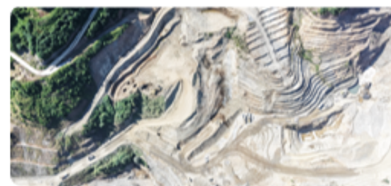
Construction of the structural dam in the Karatza Lakkos Valley
