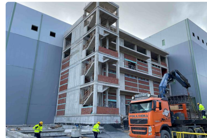
Process control building
