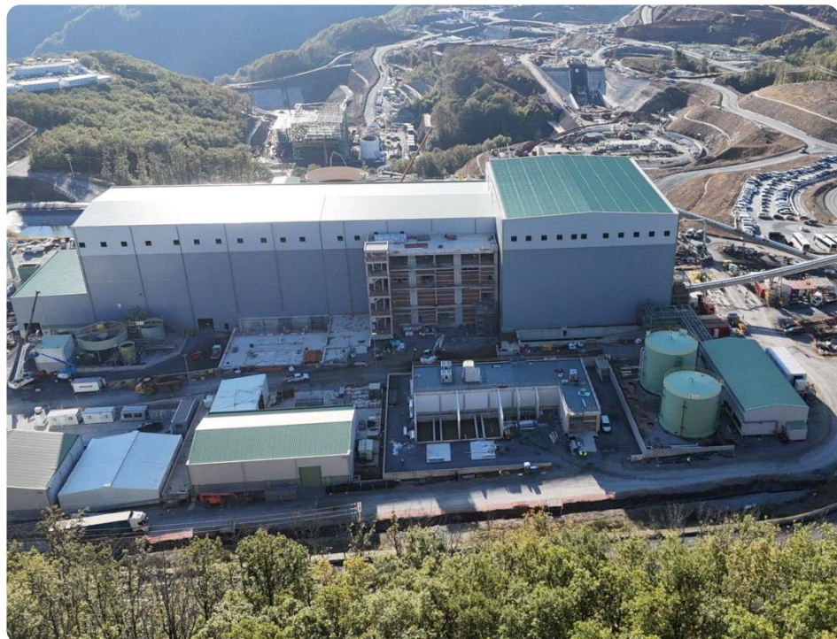
Process plant overview
