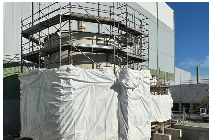
Stand up of the guar building
