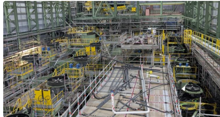
Flotation area piping and cable installation
