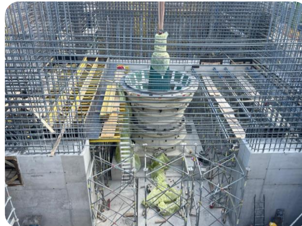
September 2025: Top photos: Primary Crusher top and bottom shell installation completed. Bottom photos: Main shaft installation completed and final components
