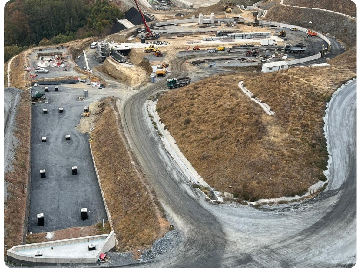
September 2025 – Concrete pedestals for the conveyors that will transport ore from the coarse ore stockpile to the processing plant (concentrator)
