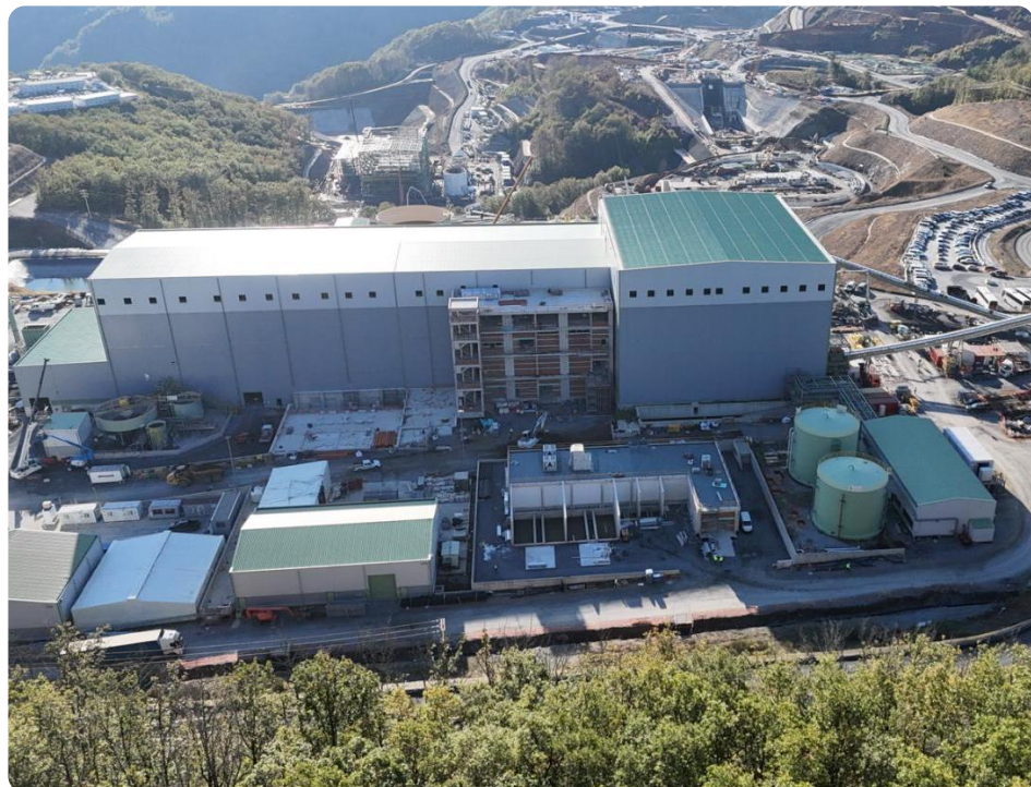
Process plant overview
