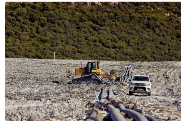
Deep ripping system
