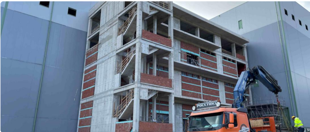
Process control building
