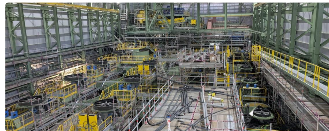
Flotation Area Piping and Cable Installation
