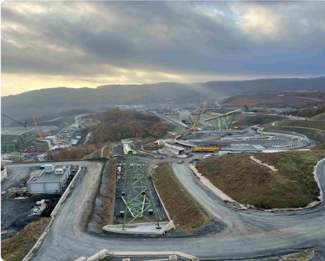
SAG feed conveyor and coarse ore stockpile dome
