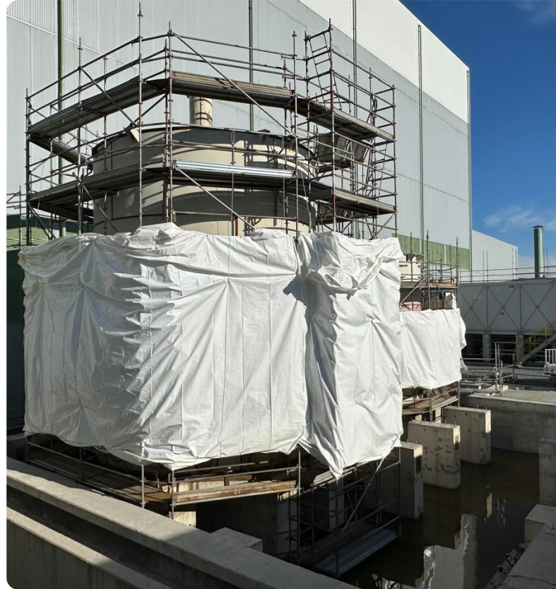
Guar building tank erection
