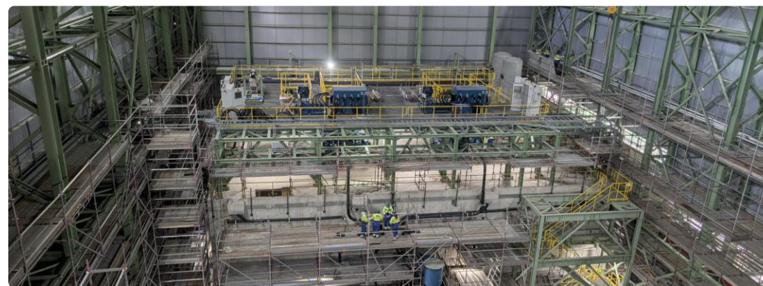
Concentrate Filter Press Piping Installations
