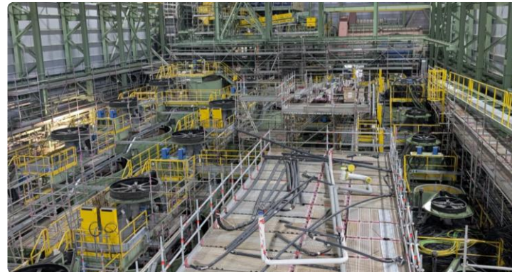
Flotation area piping and cable installation
