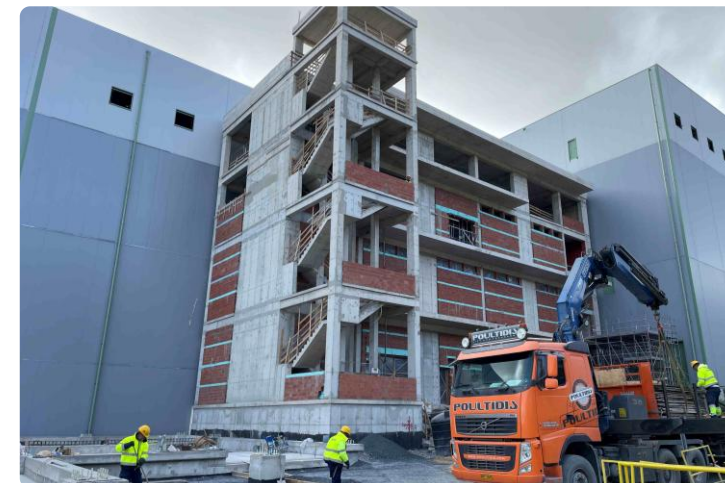
Process control building
