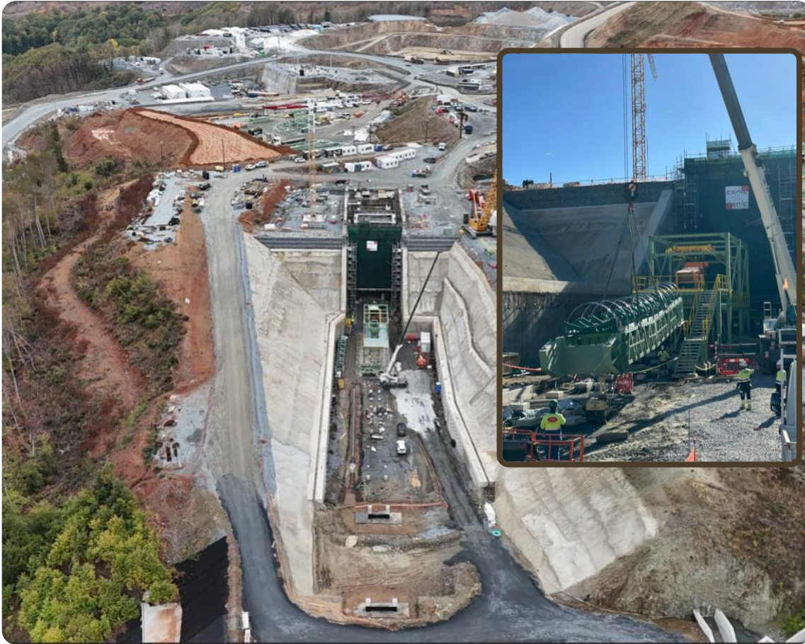
Primary crusher overview. Top right insert – closer up view of conveyor preassembly.
