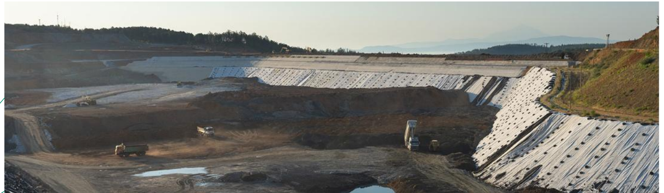
Kokkinolakkas filtered tailings facility
