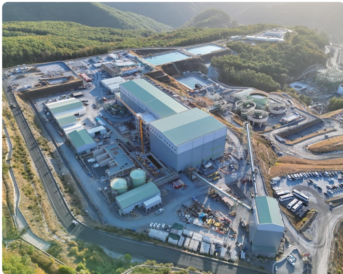
Aerial – process plant
