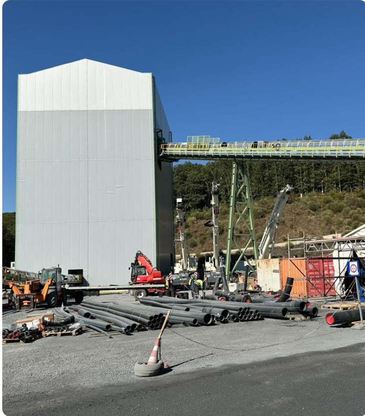
Pebble crusher building
