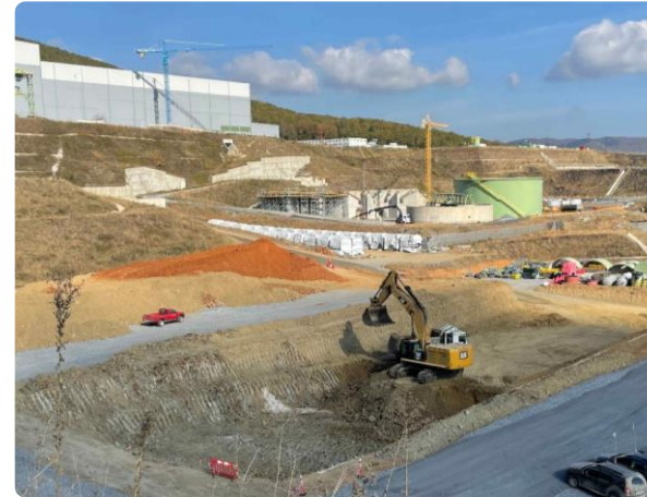
Course ore stockpile – reclaim feed excavation
