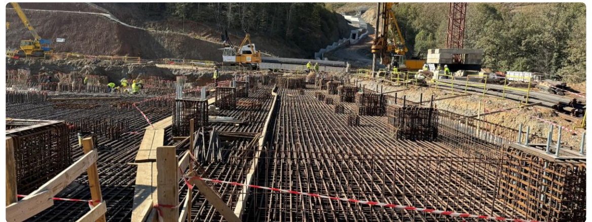
Filtered tailings building – close-up view of the piling
