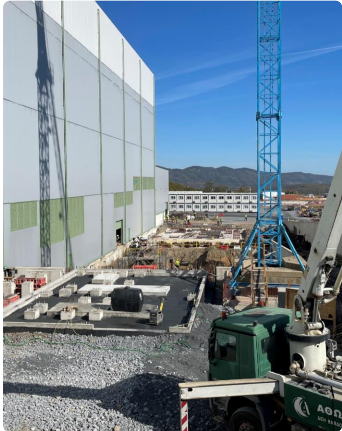
East side of main process plant building
