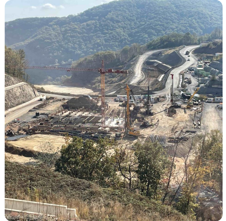
Three active drills are working at the filtered tailings facility, where 388 piles have been completed out of a total of 871. All piles for the filtered tailings building have been completed.
