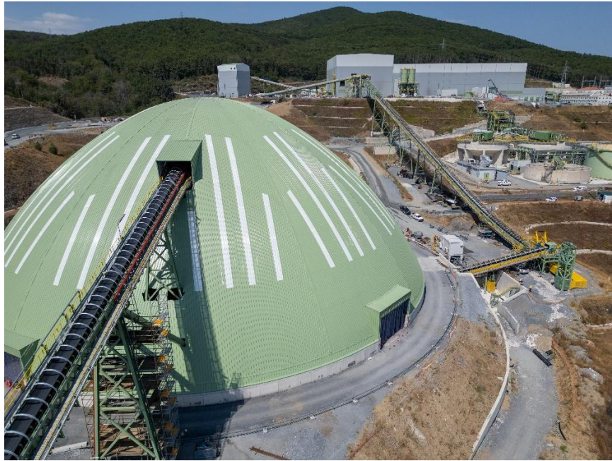
Stockpile dome and process plant
