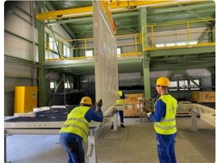
Filter Press Pre-Assembly
