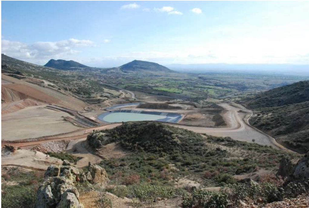
Figure 19-6: Rock Dump Collection Ponds
