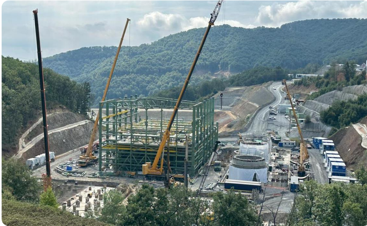
Filtered tailings plant facility overview, with tank farm progressing on the right and the foundation of the compressor building on the left
