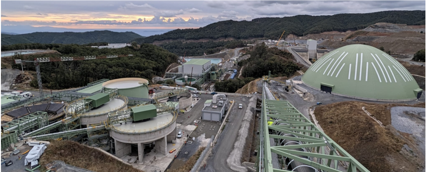
View of coarse ore stockpile dome (right), thickeners (left), filtered tailings building (background)
