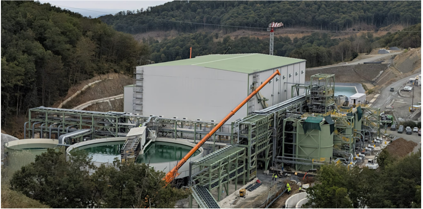
Filtered Tailings Facility
