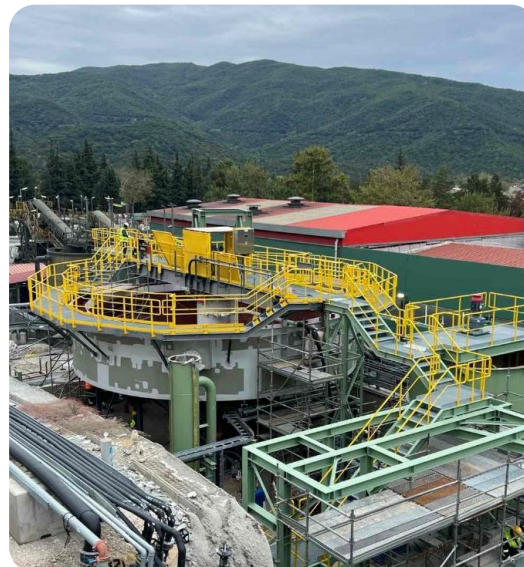
From L-R: Au Thickener: Steel structure erection; Au Thickener: Installation of bridge and rake mechanism; VTM: Mechanical works.
