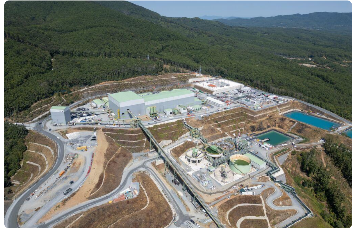
Aerial of site, Skouries
