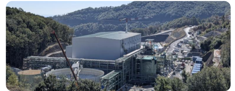
Tailings filter area
