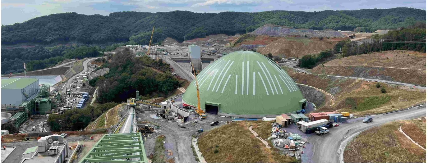
Coarse ore stockpile dome
