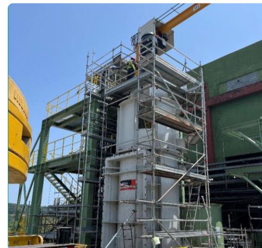
Verti-mill installation works
