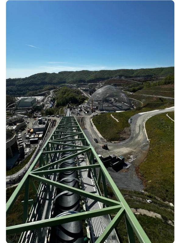
SAG Mill conveyor, Skouries
