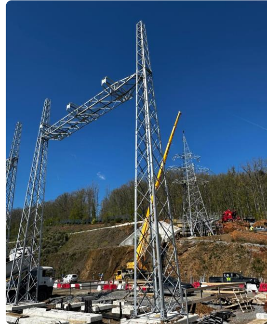
Tower 11 assembled & erected
