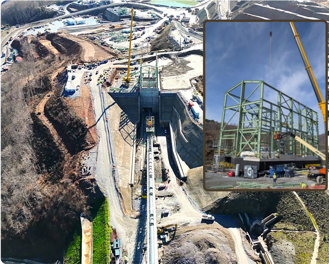
Primary crusher overview. Top right insert – closer up view of primary crusher building erection.
