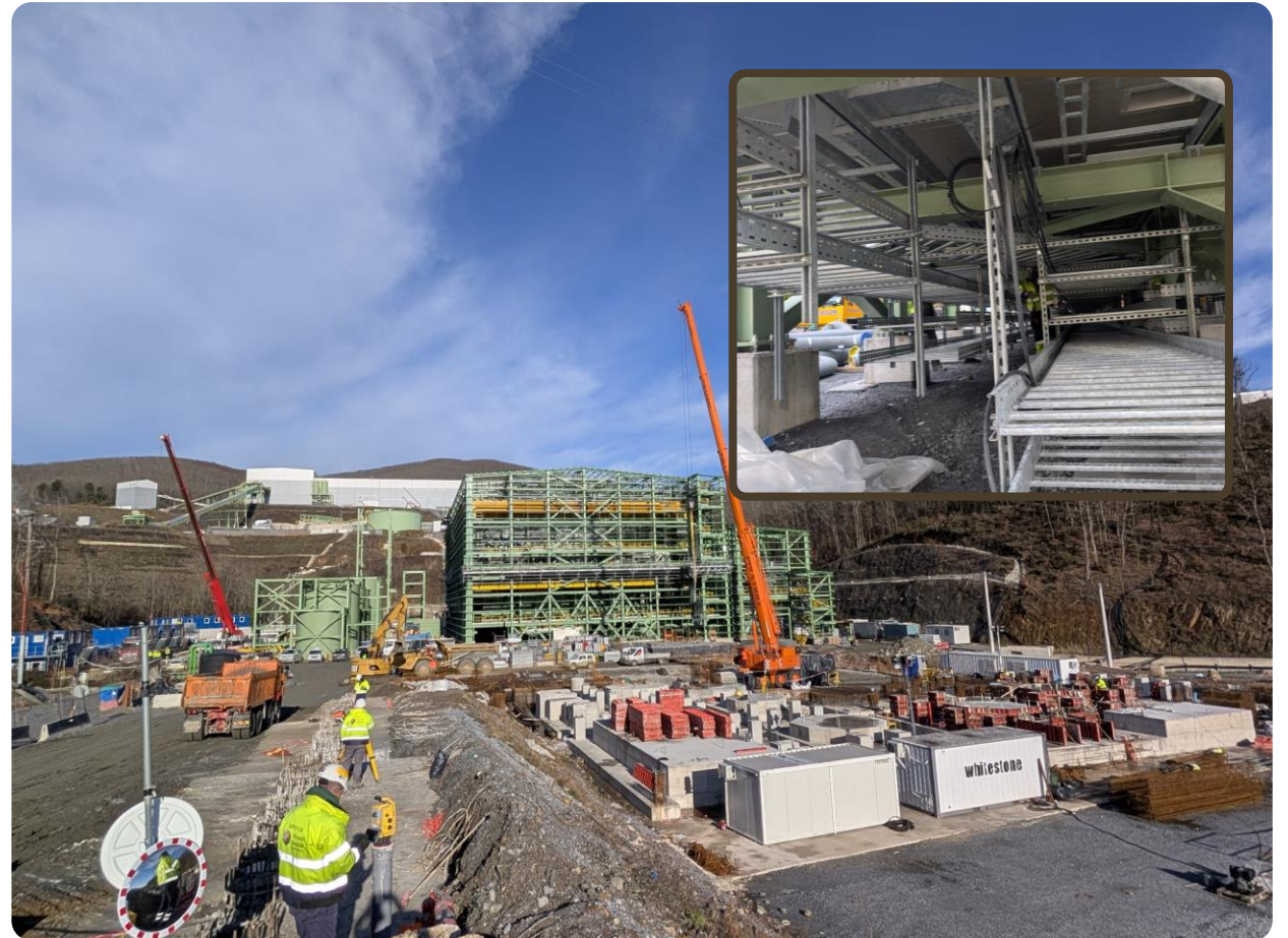
Tailings filter press building. Top right insert – closer up view of first cables being pulled.
