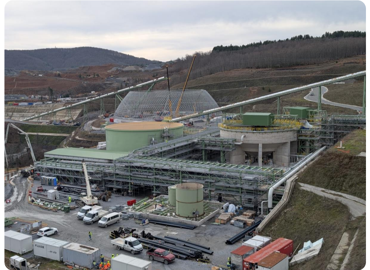
Tailing thickener pipe rack and distribution box
