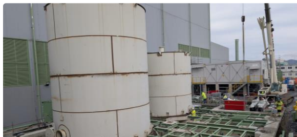
Guar elevated floor erection
