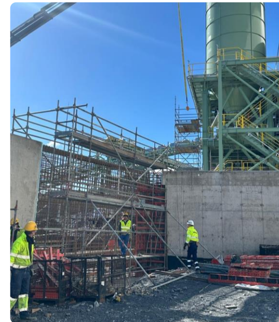
Lime building area – retaining wall construction
