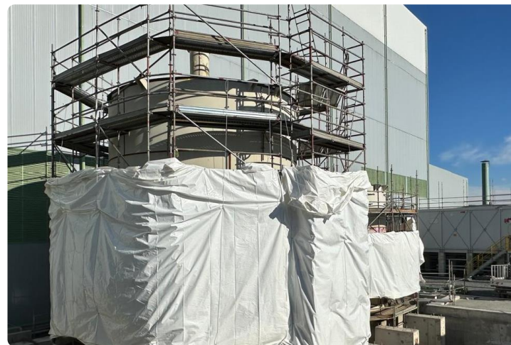
Stand up of the guar building
