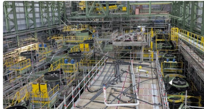
Flotation area piping and cable installation
