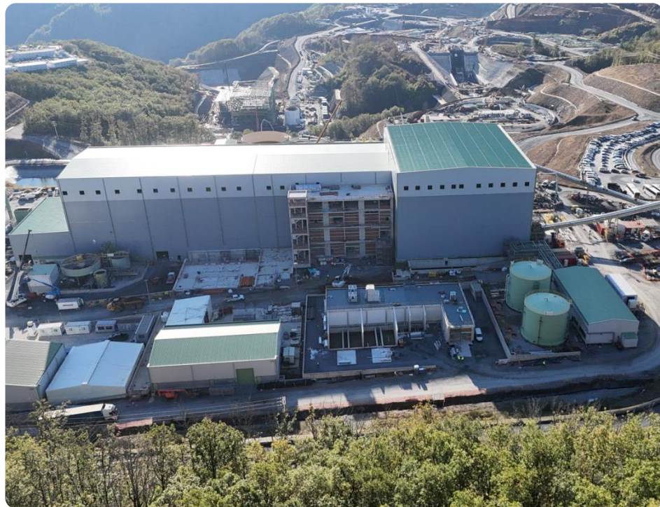
Process plant overview
