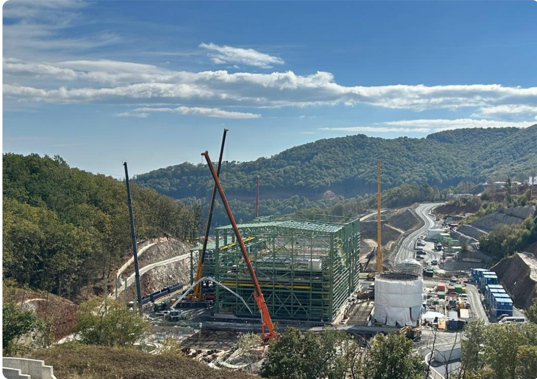
Filtered tailings plant overview, with tank farm progressing on the right and the foundation of the compressor building on the left
