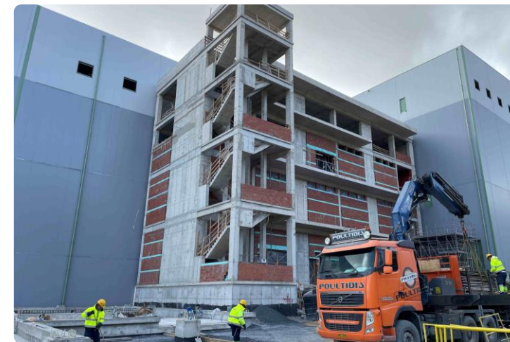
Process control building
