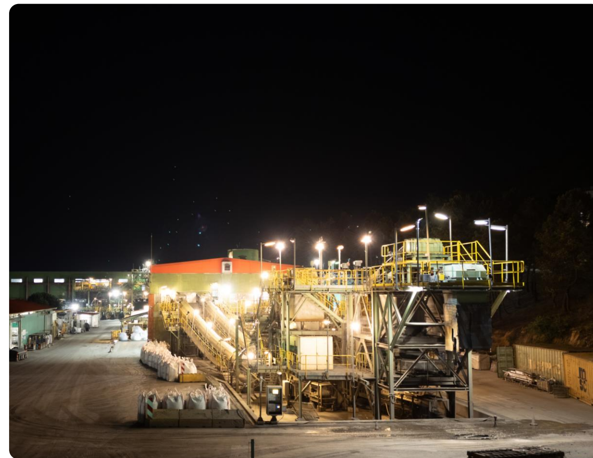
Olympias – mill and concentrate load out area.
