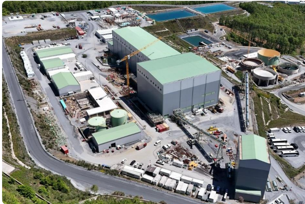
Process plant overview
