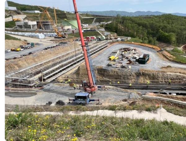
Course ore stockpile – reclaim feed tunnel
