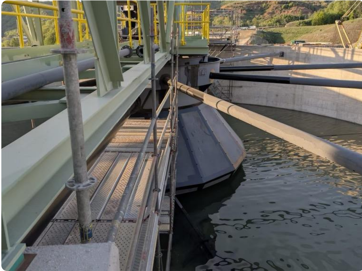
Tailings thickener circuit - water testing commenced in clarifier.
