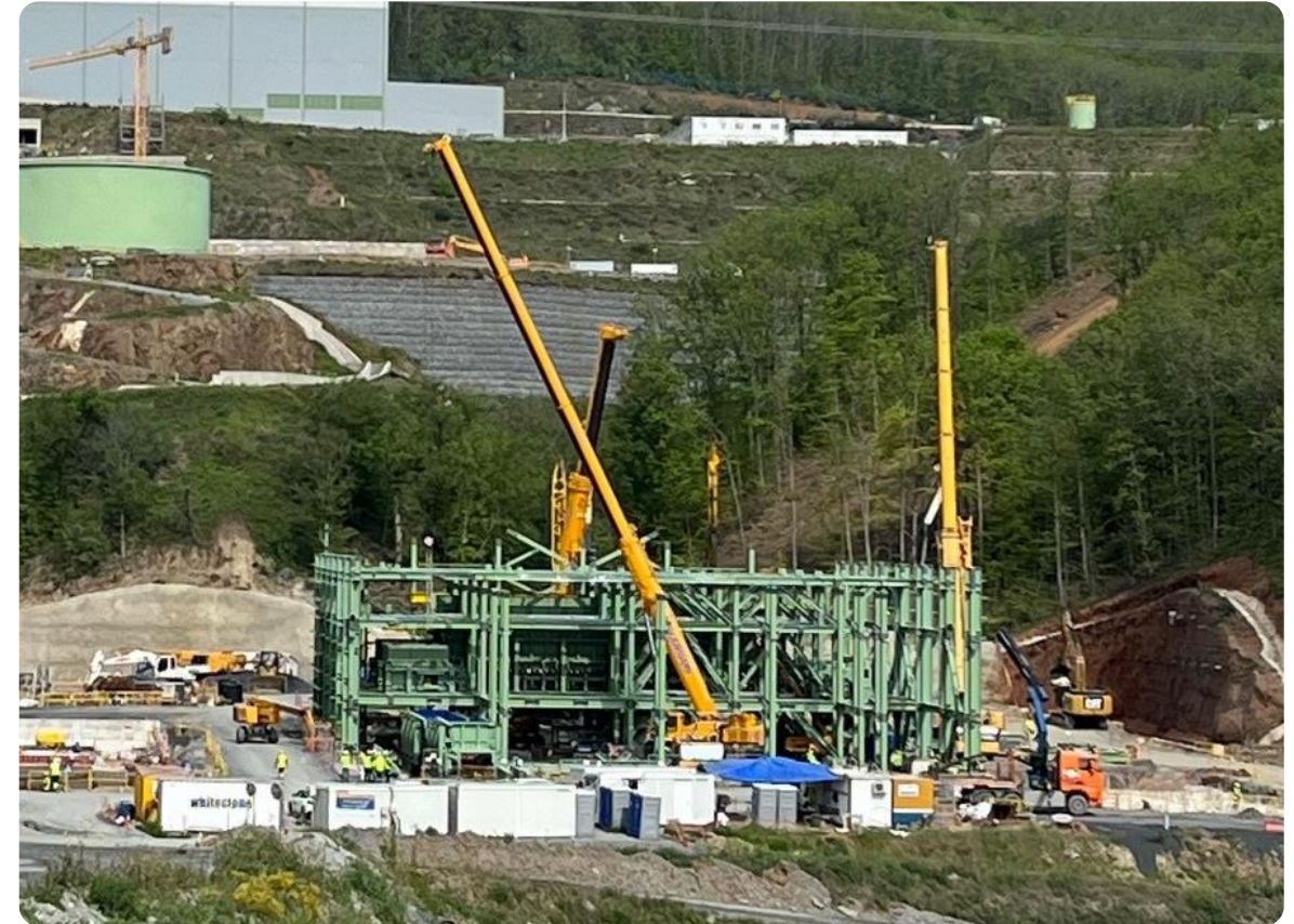
Filtered tailings building
