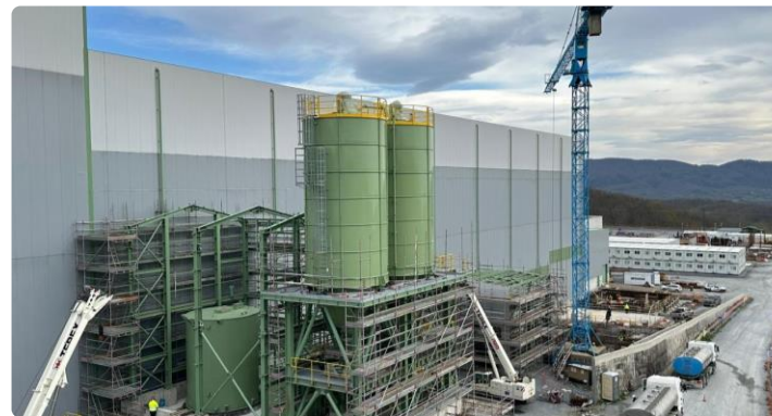
Lime plant building construction
