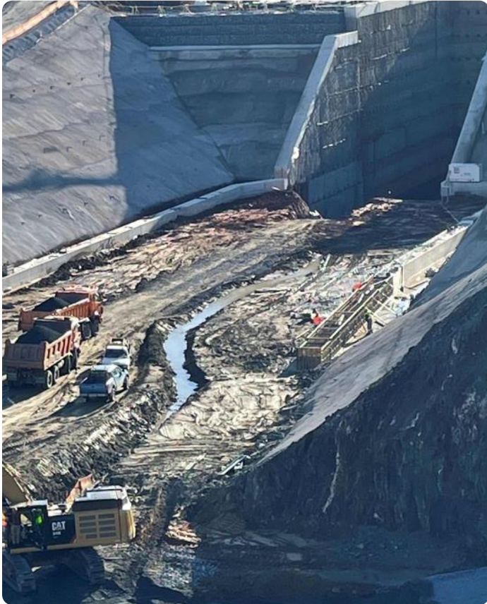
Primary crusher overview
