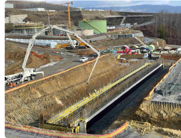
Course ore stockpile – reclaim feed tunnel
