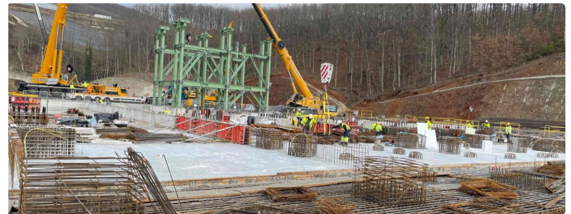
Filtered tailings building – close-up view of the completed piling
