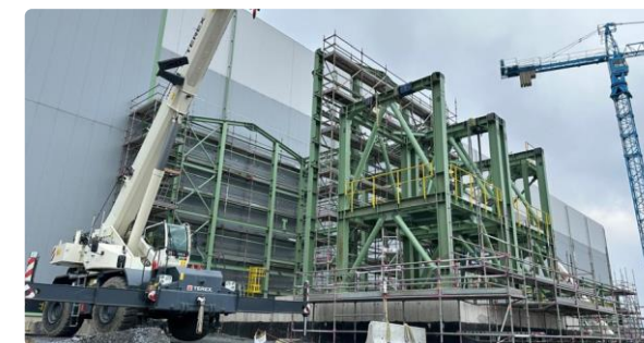
Lime plant building construction
