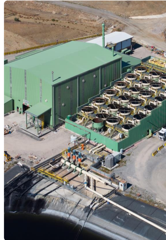
North-ADR plant at Kışladağ completed.
