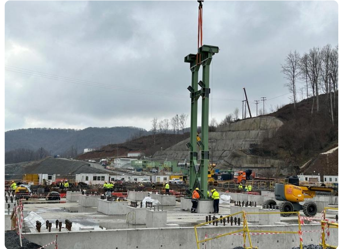
Filter plant – first structural steel installation – February 8, 2025
