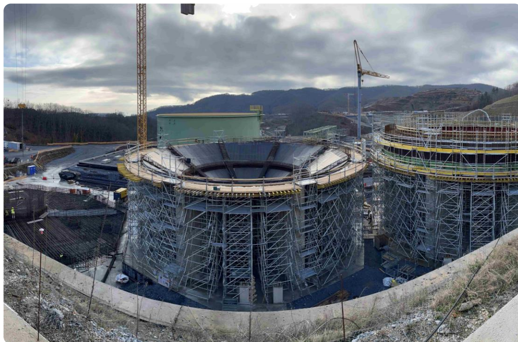
Thickeners – concrete works progressing on first two, and construction on third thickener has commenced.
