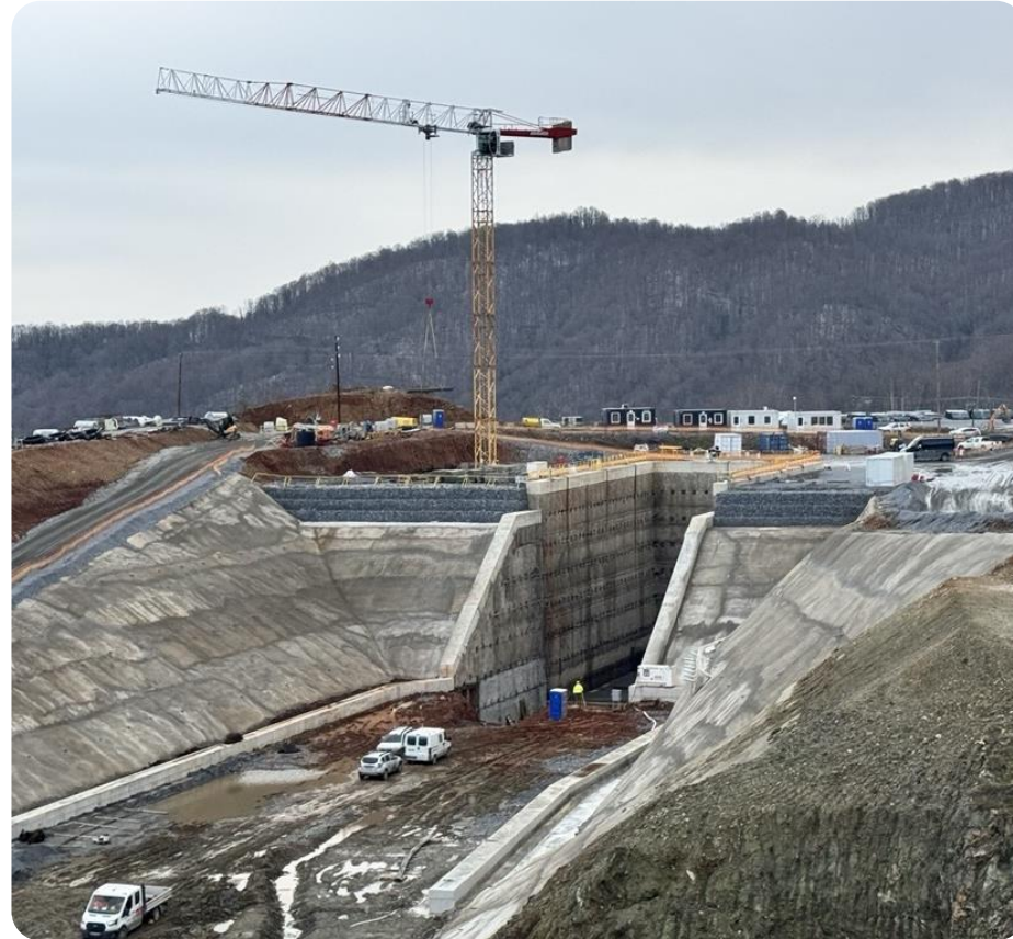
Fixed location construction crane
