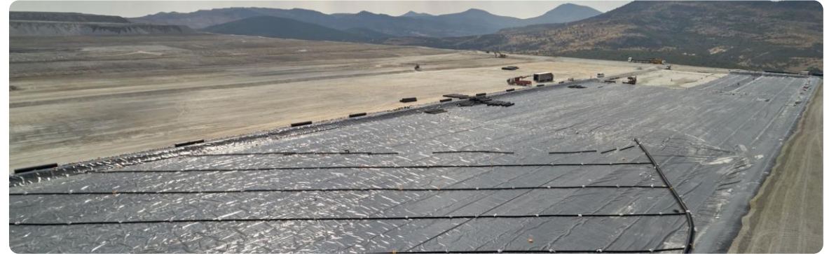
Inter-lift liner placed at various levels
