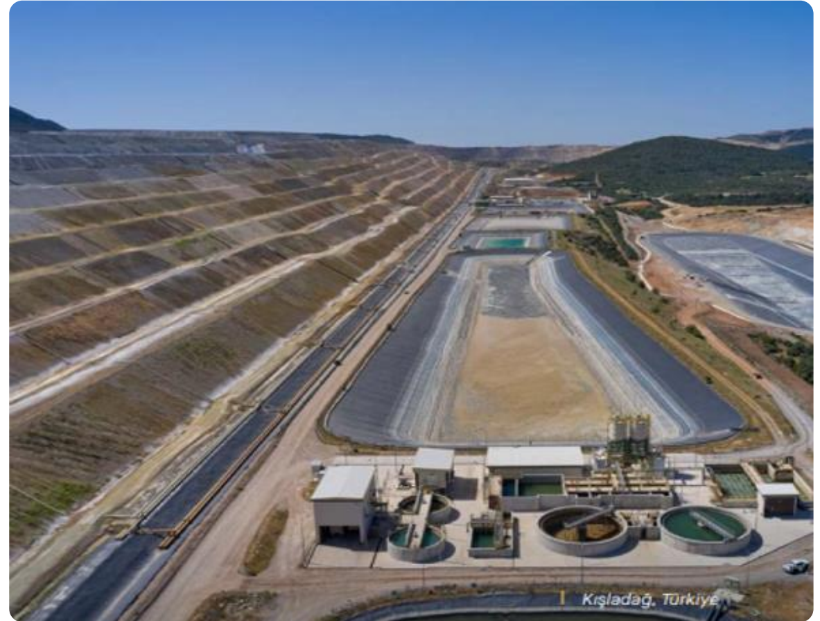
Heap leach process solution ponds (located external to South Heap Leach Pad)
