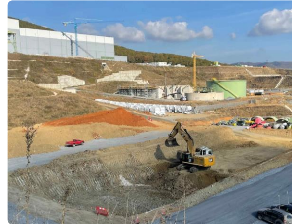
Course ore stockpile – reclaim feed excavation.
