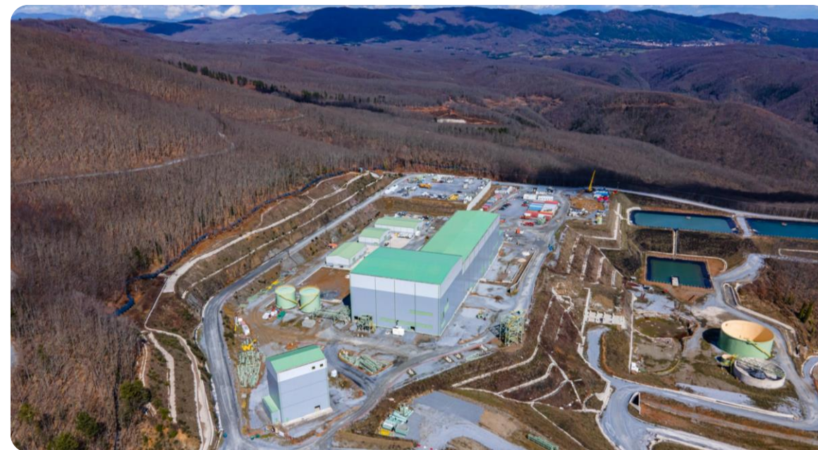
Aerial view of the mill building at Skouries.
