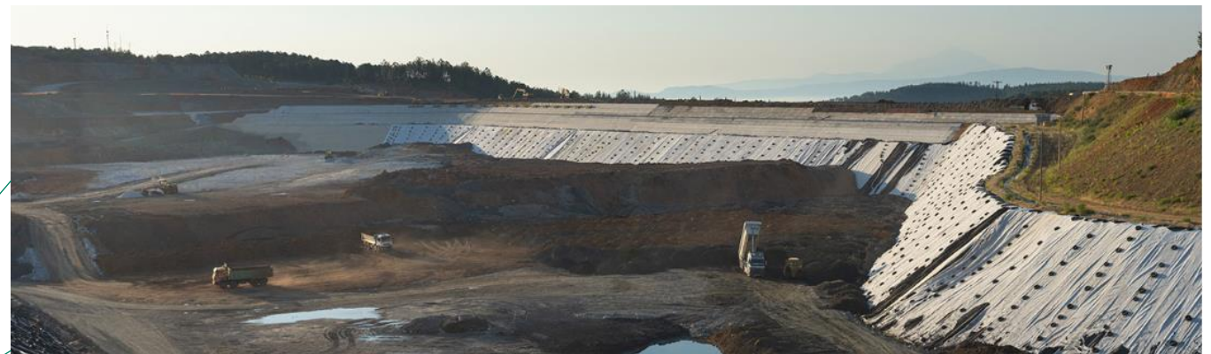
Kokkinolakkas dry-stack tailings facility
