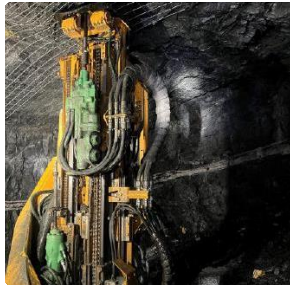
Infill drilling at Ormaque
